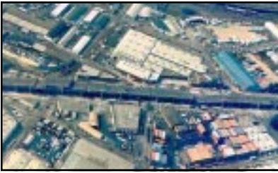
The collapsed section of the Nimitz Freeway.
